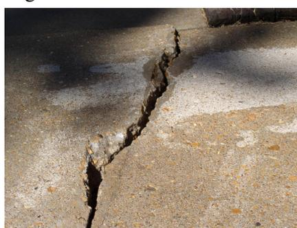
Cracked slabs brought up to level and repaired with ShurBond 550 Epoxy Adhesive and ShurBond 100 Polymer Concrete. Picture on the right also shows severely spalled area
