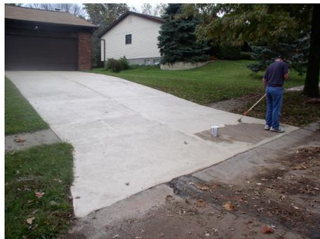
Repaired and removed major trip hazard at crack closest to the sidewalk. Repaired major cracks in driveway and severed spalled area. Application will add many good years of service to the driveway.
