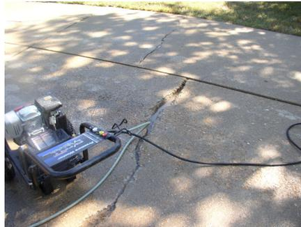
Cracks prepared by grinding and power washing.
