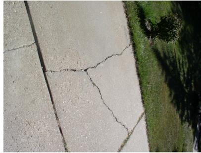
High Pressure Water Blast Actually done twice (first to just clean surface and cracks and then after grinding cracks etc.)
