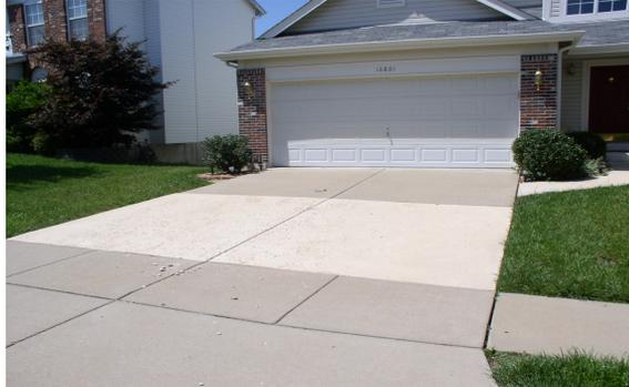
Spalled areas are repaired and protected from further spalling and entire driveway is uniform in color.
