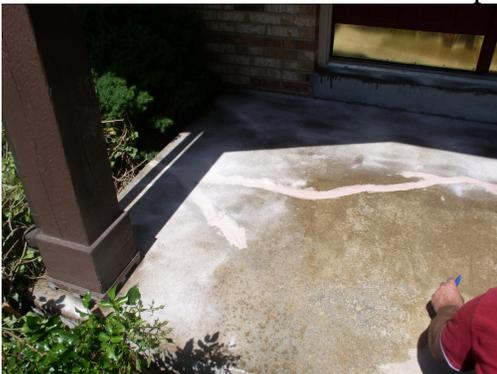
STEP 2. ShurBond 550 liquid was applied to the entire surface and while wet crystal sand was broadcast to rejection and the system allowed to cure and then the excess crystal is removed.
