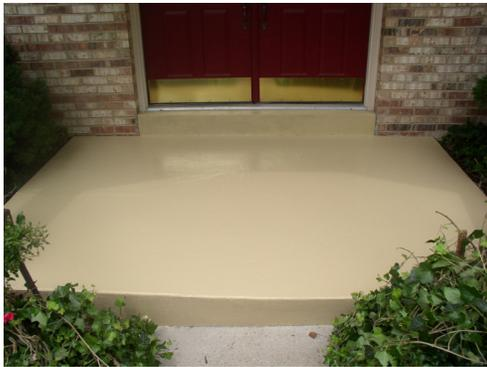
The after the result upon completion. The surface is repaired and sealed and the finished product is easy to clean and is non-slip when wet or dry. The same process us used on a driveway, sidewalk, patio or porch with the same results.
