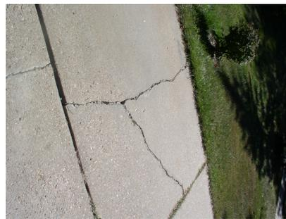
STEP 2 Clean the surface deep into the cracks and expansion joints.
