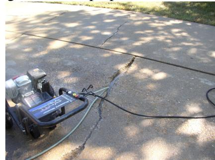
Cracks prepared by grinding and power washing.
