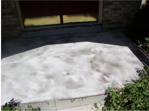
The final step is to apply the WOHL Concrete Color Stain to the surface.
